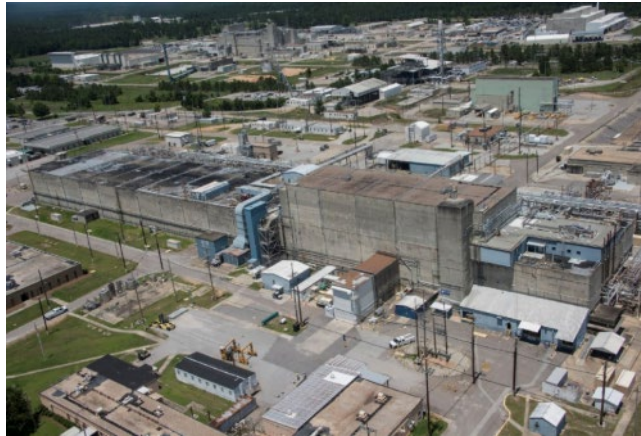
H-Canyon Processing Facility
