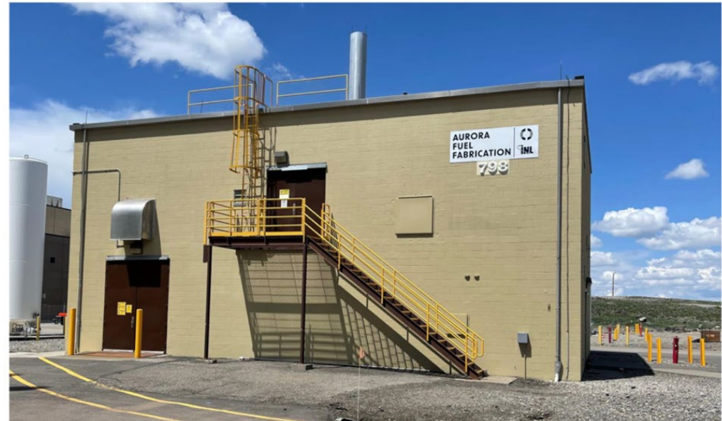
Pre-decontamination and decommissioning view of MFC-798
