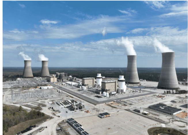
Figure 2 Plant Vogtle in Waynesboro, Georgia Office of Nuclear Energy (81)
