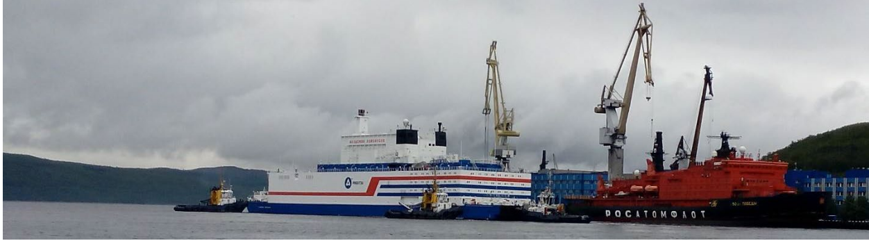
Figure 24: The Russian Floating Nuclear Power Station Being Transported from Murmansk (78).
