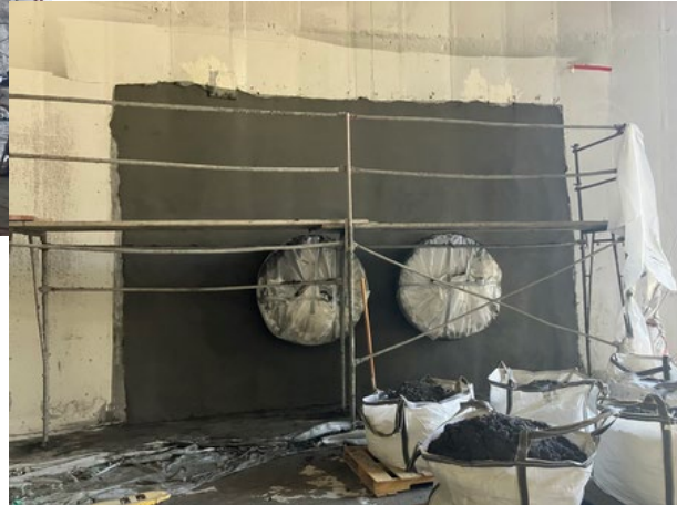
DOME developer penetration with shotcrete in place
