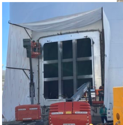
DOME hatch welding
