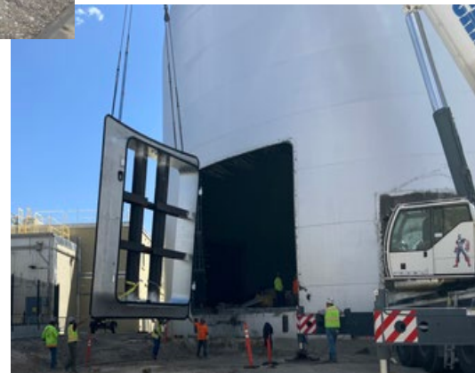
DOME hatch cutting and fit up
