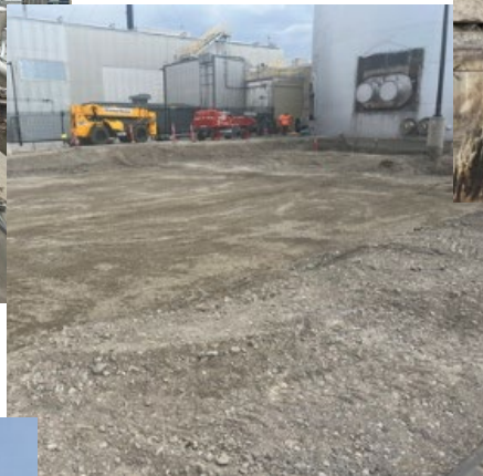
Yard grading at DOME site
