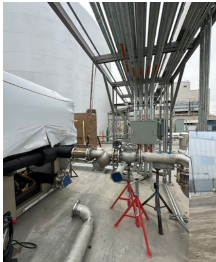
DOME utility installation
