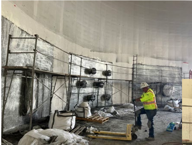
DOME penetrations with unfinished shotcrete in place
