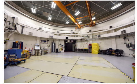
The 50-foot diameter cell provides space for small experimental reactor demonstrations.
