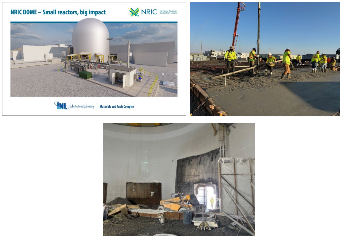
Figure 4 DOME construction photos
