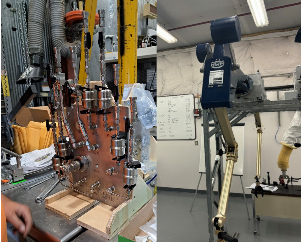
Figure 17 Photographs of manipulators at INL and a feed-through ready for installation.
