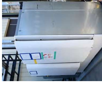
Bloom Energy 100 kWe HTE Stack Module
