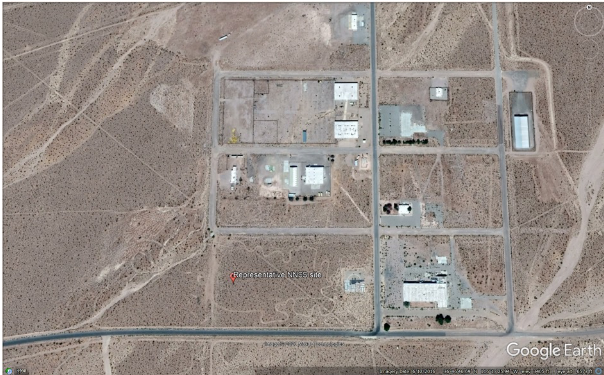
Figure 6-28: NNSS Representative Site. Central point for model analysis of siting attributes is shown at the pin drop near the lower center area of the image.
