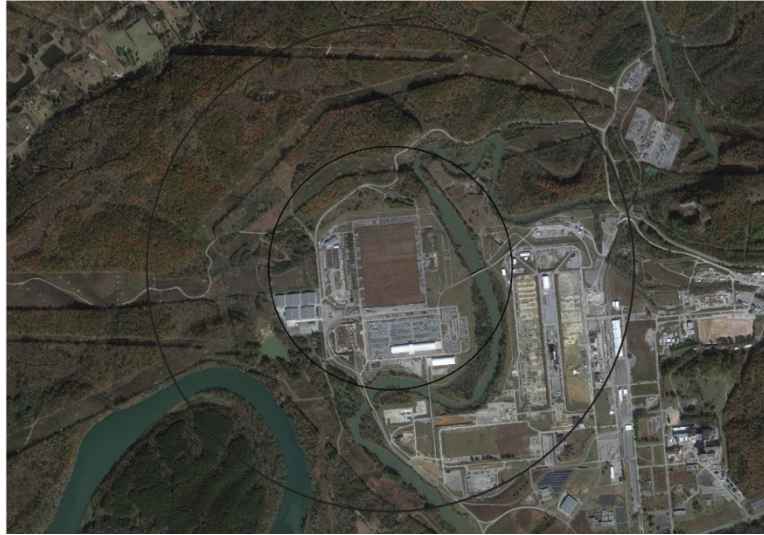
Figure 6-52: The ETTP OR-SAGE results for population density, safe shutdown earthquake, faults, streamflow, protected lands, and proximity to hazards indicate no query threshold issues.
