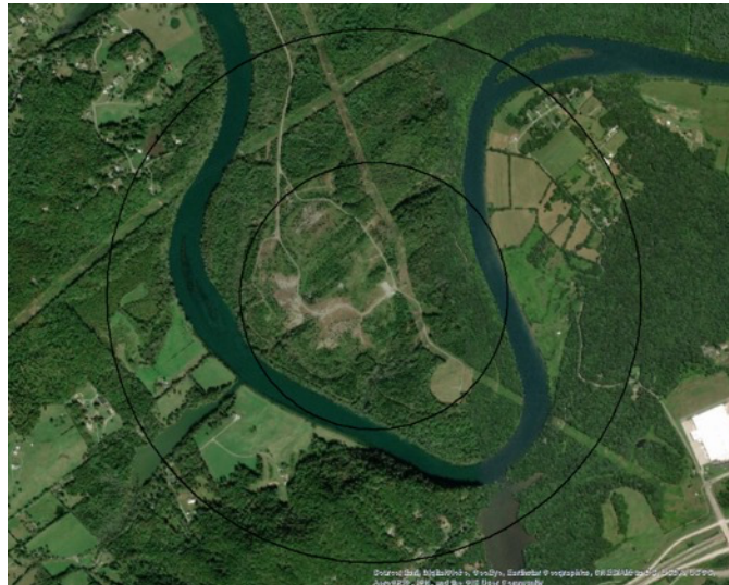
Figure 6-46: TVA Clinch River OR-SAGE results for population density, safe shutdown earthquake, faults, streamflow, landslide risk, and proximity to hazards indicate no query threshold issues.
