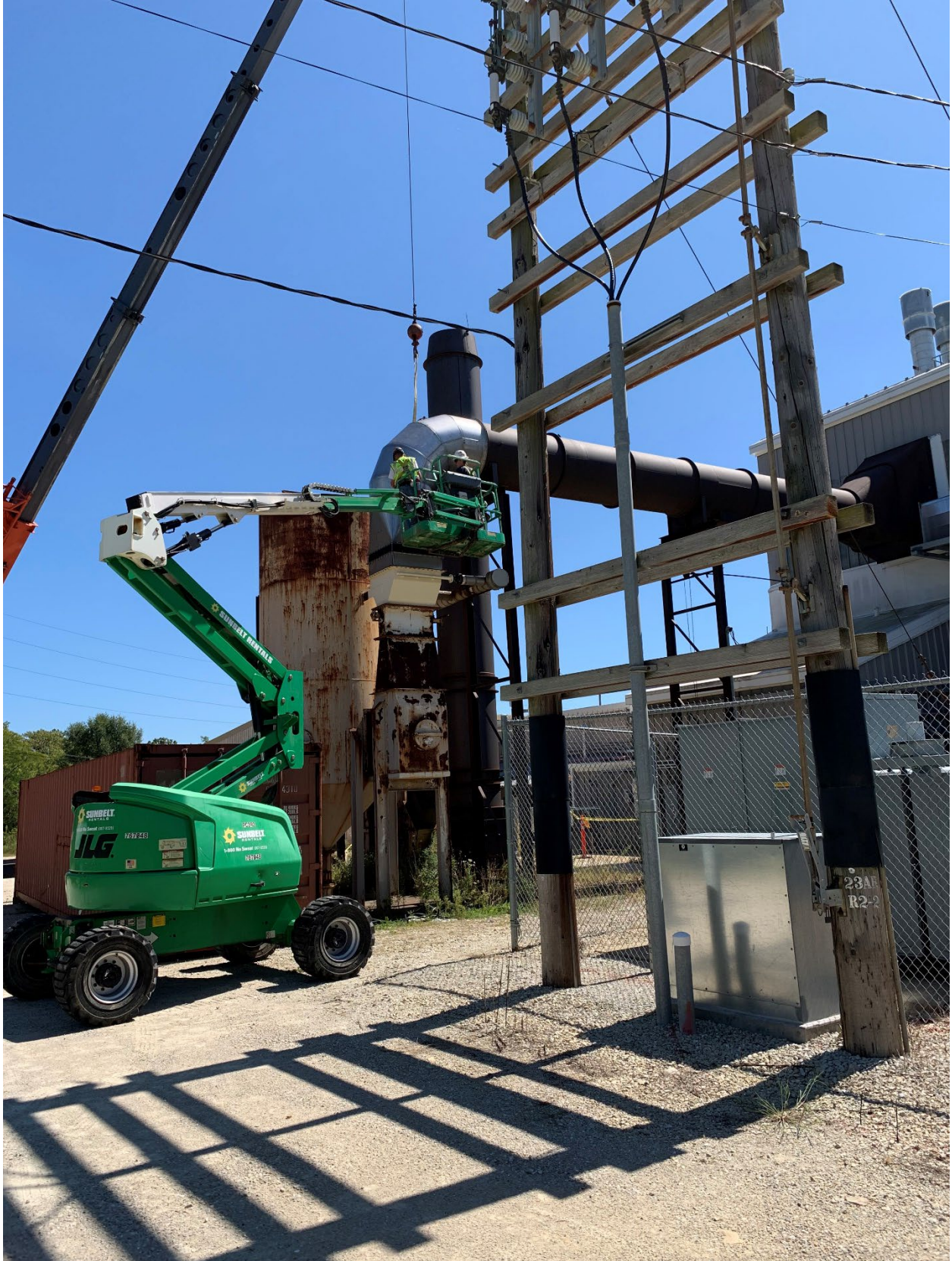
Figure 26 – Construction Crew installing new ductwork
