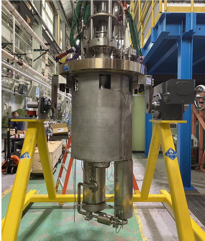
Figure 12 – THETA Following Complete Cleaning and Reassembly on the Test Stand
