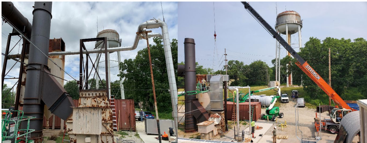
Figure 29. Ducting Removal (right) and New Stainless-Steel Ducting Installed (right).
