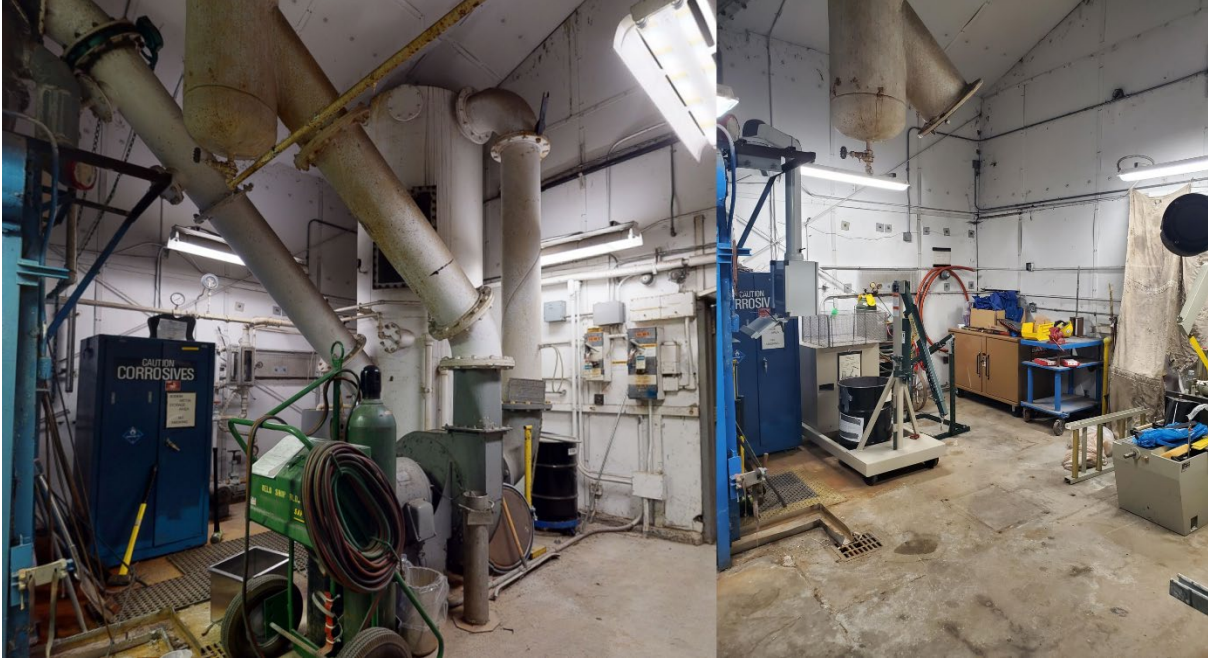
Figure 26. Room C141 Before (left) and After (right) Legacy Scrubber Removal.
